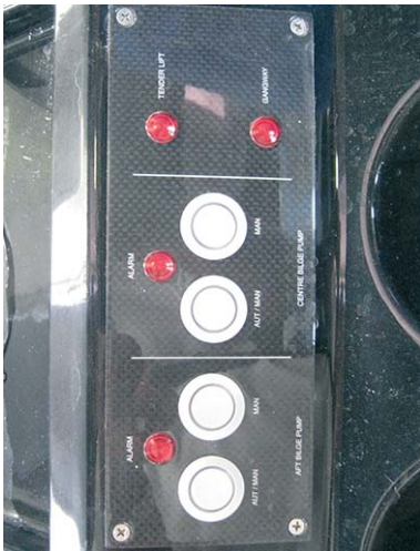
Main control station controls
