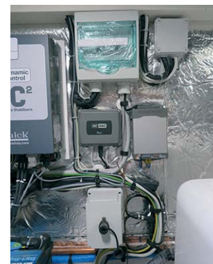
Thermal switch and battery breaker
