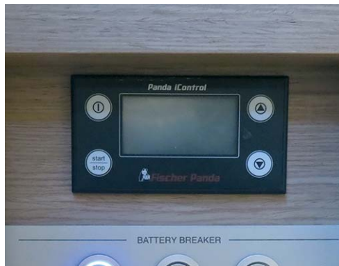
Generator control panel
