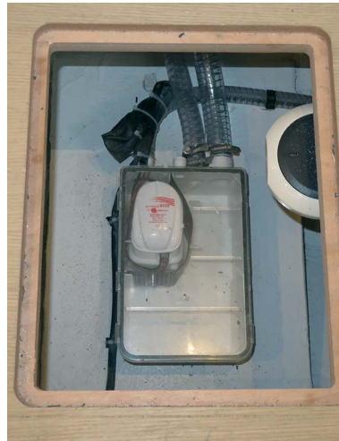
Grey water collecting tank
