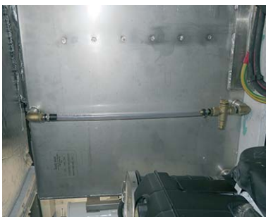
Tank visual level
