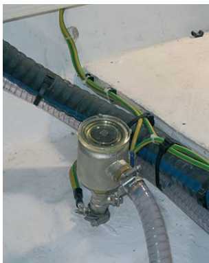
Sea intake and strainer for generator cooling
